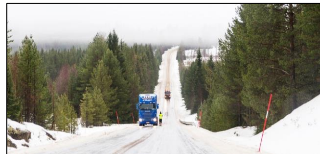
"Göteborgsbacken" prior to installation of the HHP system
