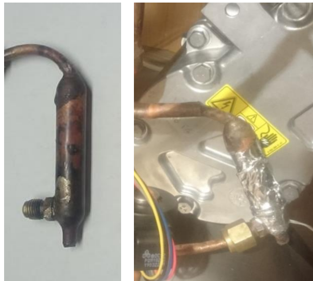
Figure 13. Filter/dryer used in Propac #1 and #2.
