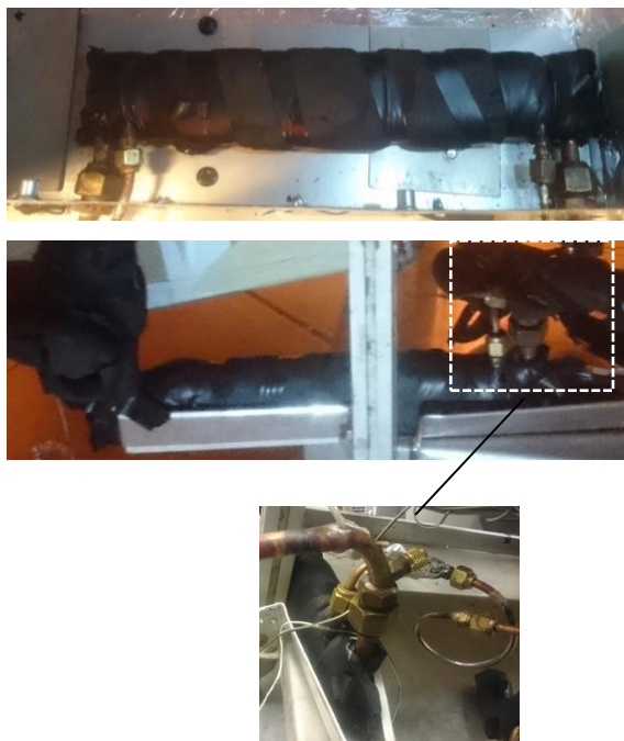
Figure 10. Internal heat exchanger orientation. Horizontal in Propac #3 (top) and vertical in Propac #1 and #2 (lower).
