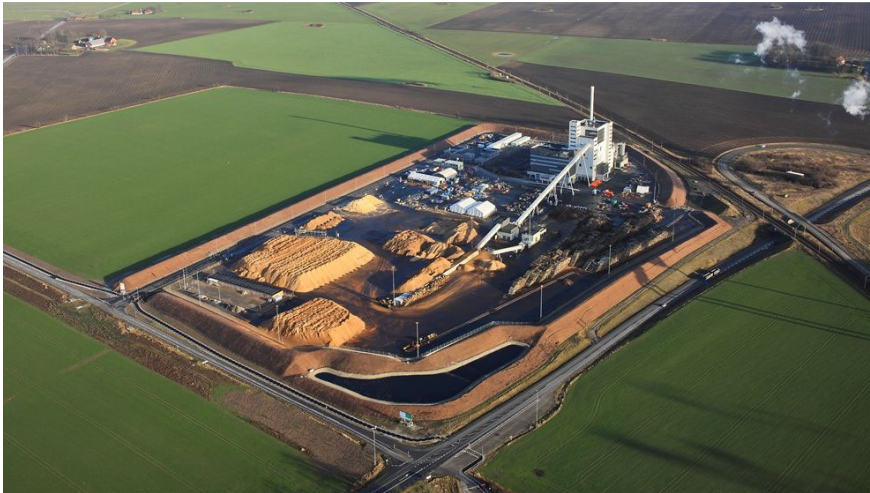
Figure 3 Overview of the Örtofta CHP plant including the biomass fuel yard.
