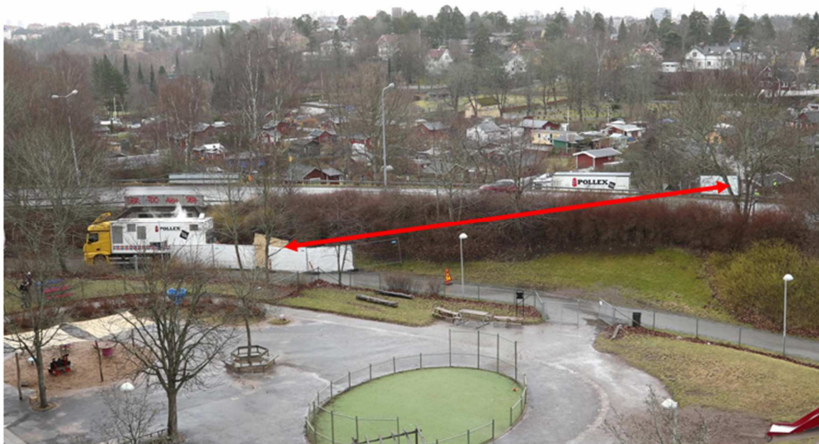
Figur 36: Installation under Rissneleden
